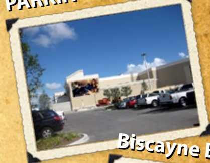
PARKING LOT WALL
